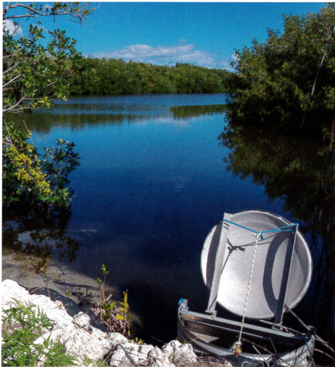
A newly installed exchange culvert at the historic mouth of Cleve Hinton Creek in Indian River Shores
