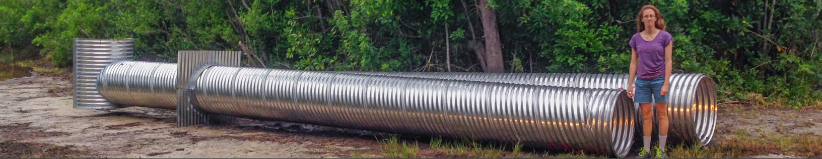
Culverts ready to be installed.
